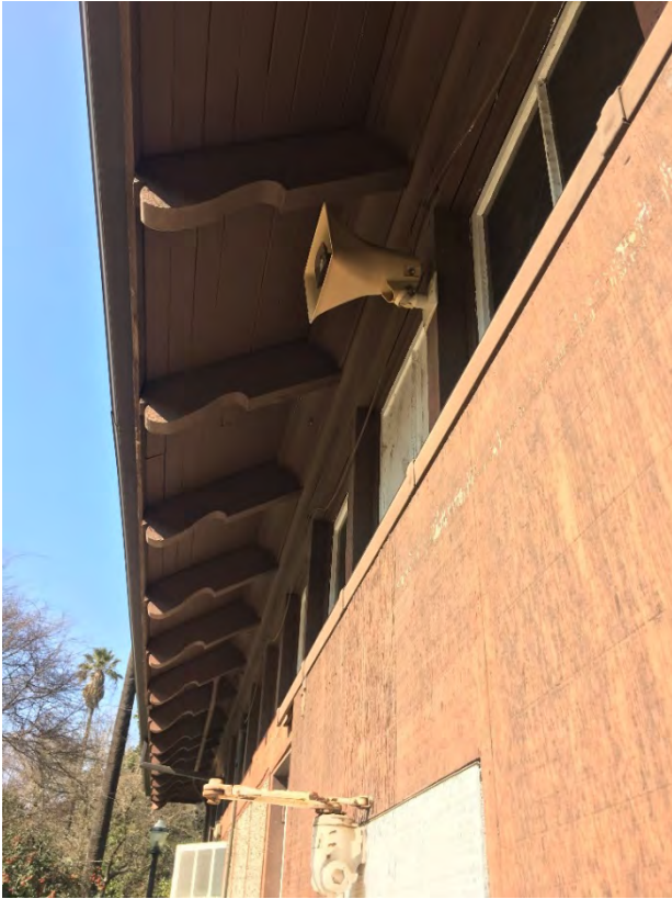
Figure 45: Typical exposed rafter tails at the exterior of the building
