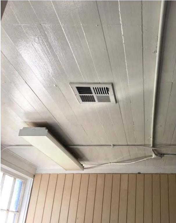
Figure 106: Ceiling lights served by rigid and flexible conduit
