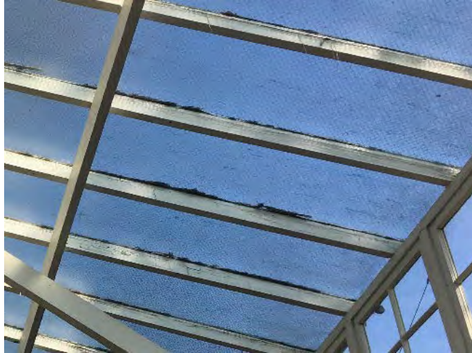
Figure 43: Enlarged view of wire glass at skylight
