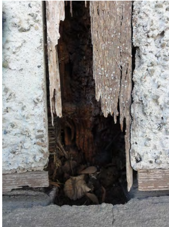
Figure 19: Base of redwood post is entirely rotted
