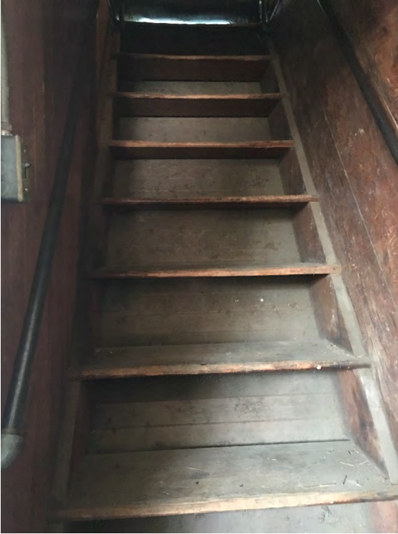
Figure 53: Attic Stair, showing 1x12 treads
