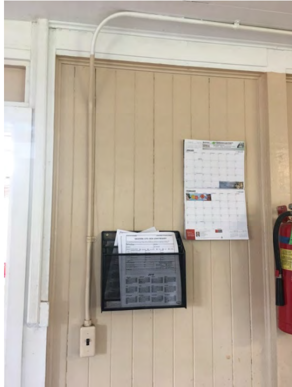
Figure 107: Light switch in former insect cage (current break room) served by surface mounted conduit
