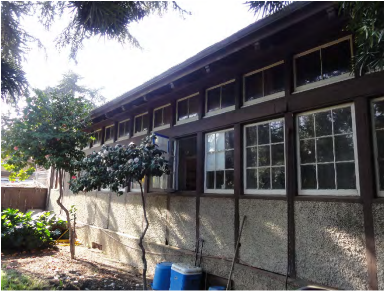
Figure 15: Rear (east) facade showing exposed posts extending from foundation to roof with windows and cement plaster panels in between.
