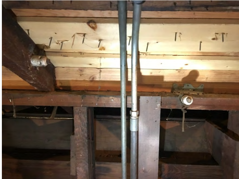
Figure 105: Abandoned knob and tube wiring still evident in the attic
