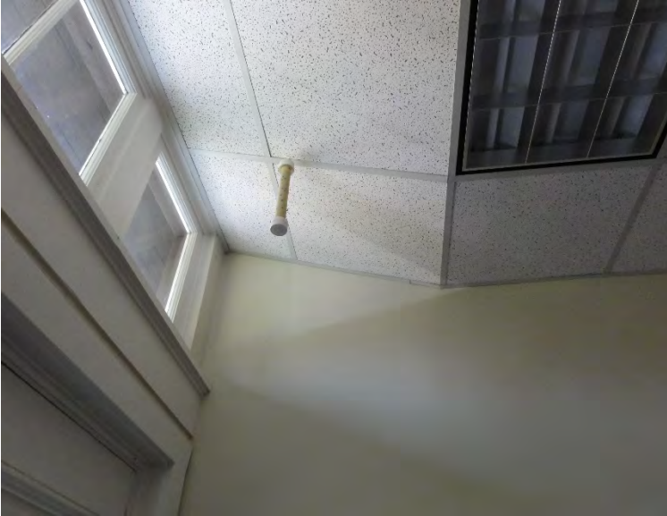
Figure 36: The original museum had higher ceilings, where the hoppers served as clerestories. The current t-bar ceiling is sloped at the exterior walls to allow the clerestories to continue to serve the main entry lobby.
