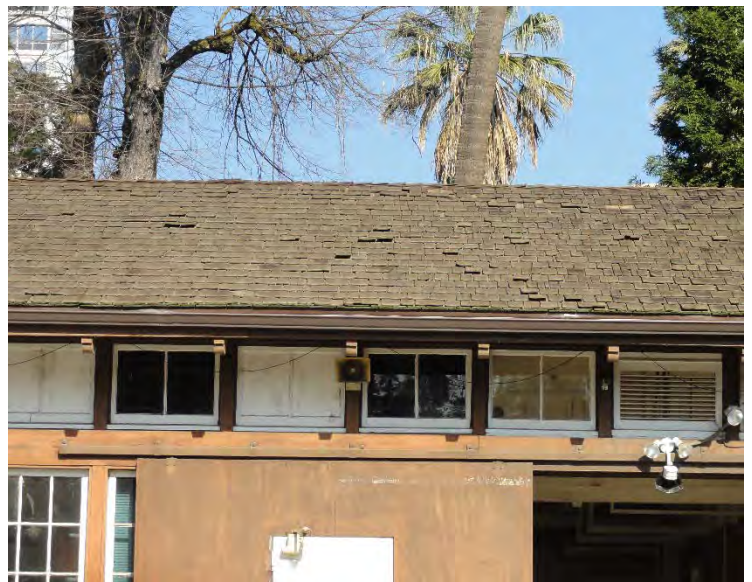
Figure 35: Three original hopper windows, two modified with painted glass and one with a louvered vent
