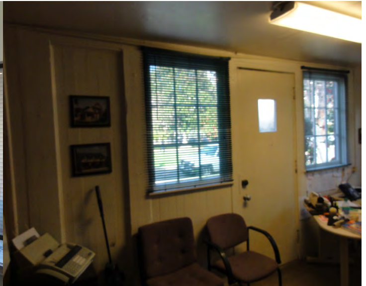
Figure 59: The exterior walls are finished in 1x3 painted redwood boards
