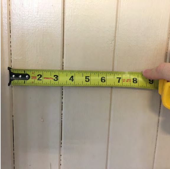
Figure 56: Painted redwood tongue and groove, typical of partitions between utility rooms on the east side of the courtyard.
