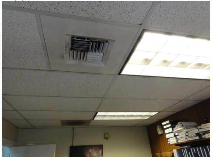
Figure 91: Supply grille can be seen in the foreground and a return air griled in the background
