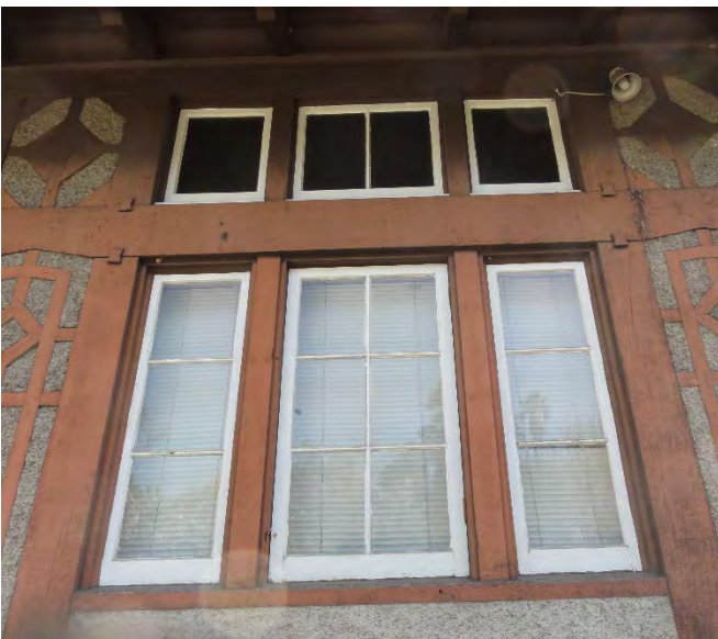
Figure 34: Three original attic hopper windows above the ground floor windows on the primary (west) façade
