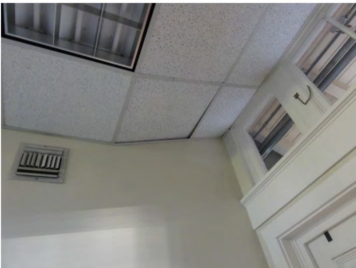
Figure 92: Supply grille located at the top of the lobby wall
