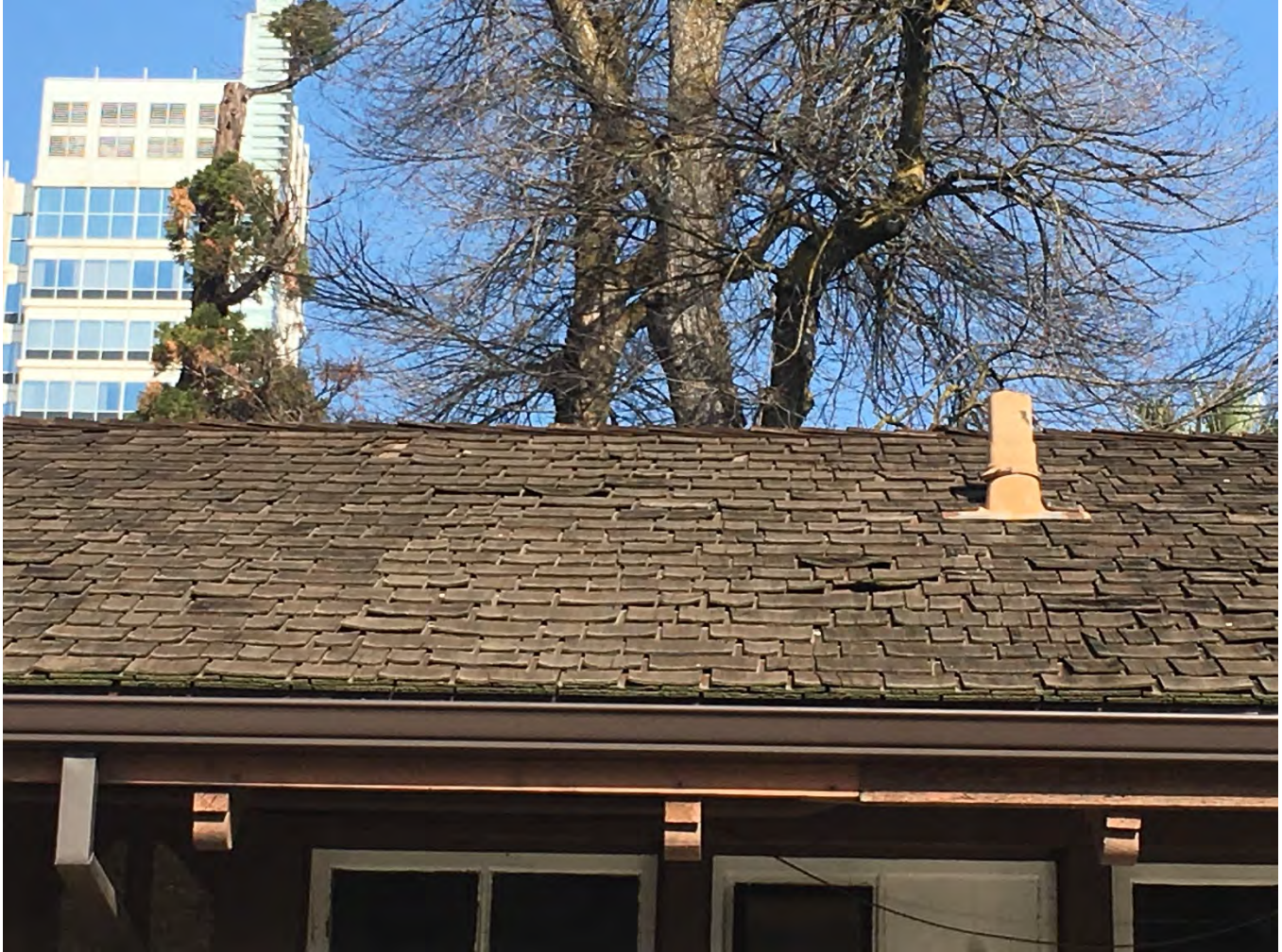
Figure 39: Close up view of shingle roof showing cupping
