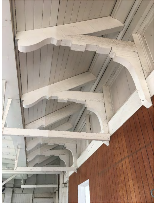
Figure 46: Typical exposed rafter tails and supporting brackets at the courtyard
