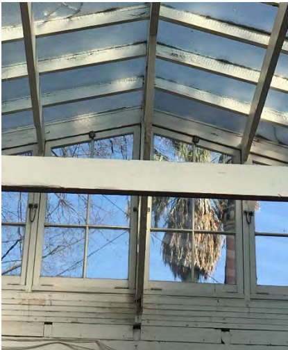
Figure 83: The vertical skylight windows are operable hoppers
