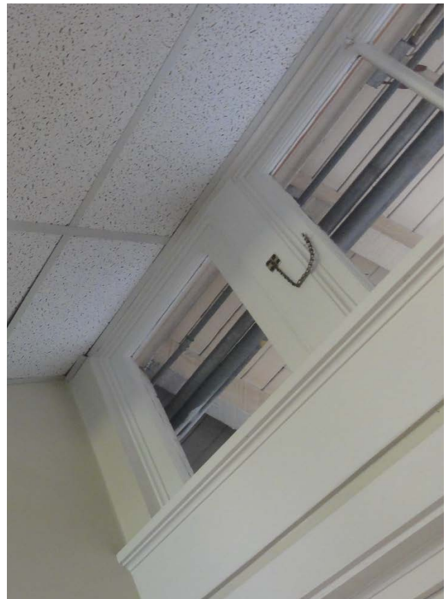
Figure 86: Typical hopper window
