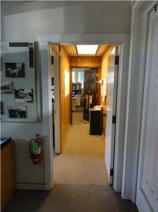
Figure 78: Simple door surround and base trim installed sometime after the 1938 remodel
