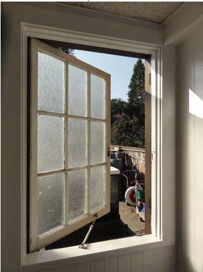
Figure 85: Typical casement window
