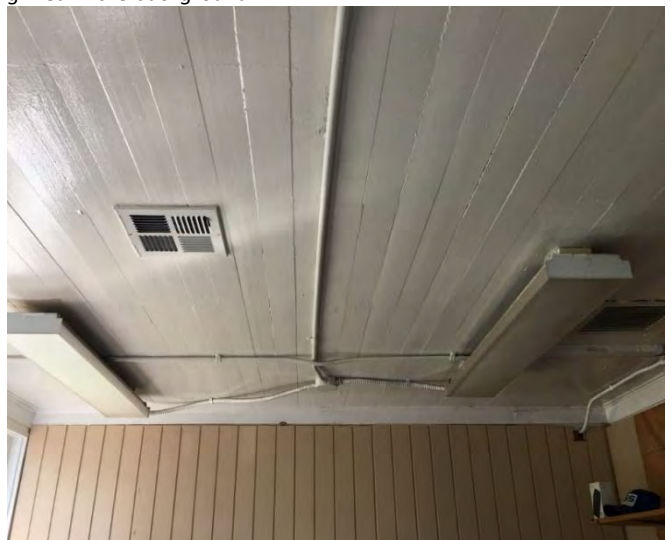
Figure 93: Another type of supply grille can be seen on the left and a return air grill on the far right
