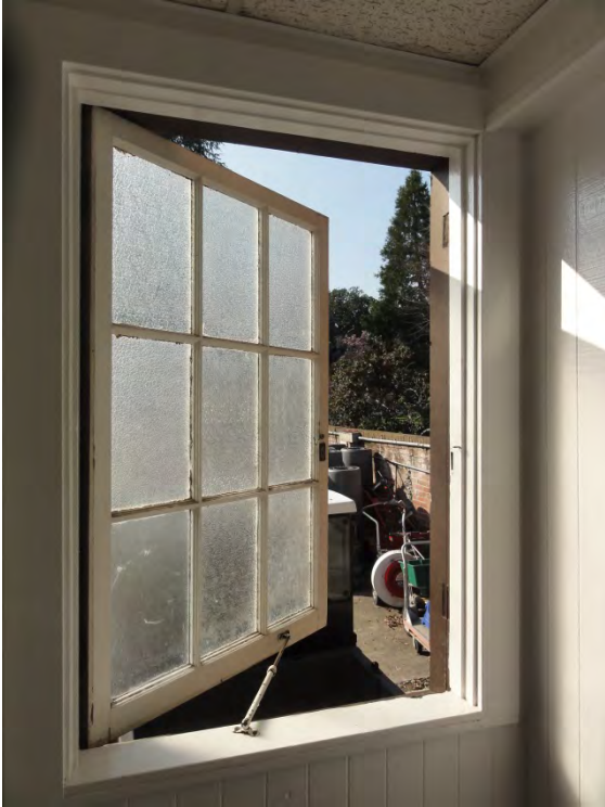
Figure 32: Interior of casement window installed in 1938
