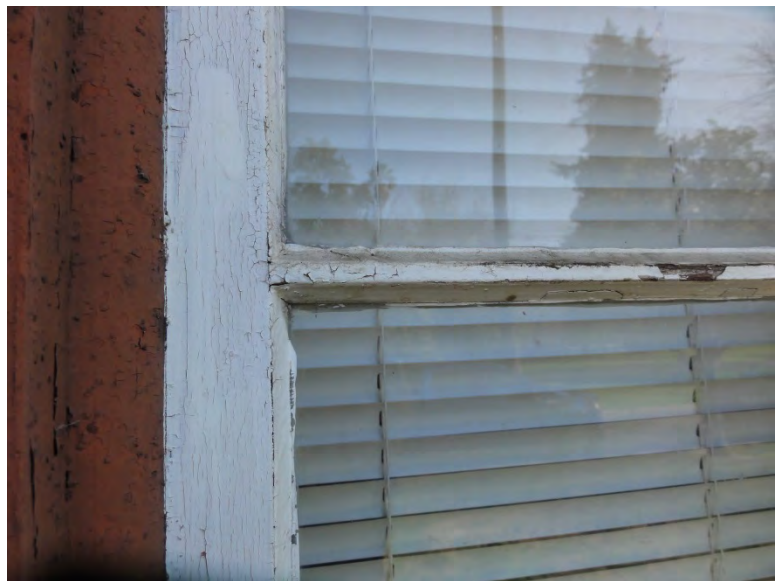
Figure 31: Detailed view of west facing window shows crazed and failing paint at the sash and muntin
