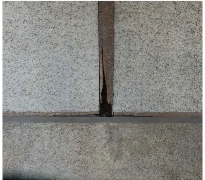
Figure 16: Base of redwood post and sill are damaged from dry rot
