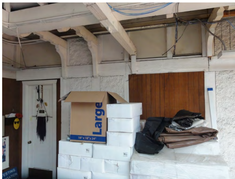
Figure 66: Courtyard cement plaster panels and redwood paneling infill
