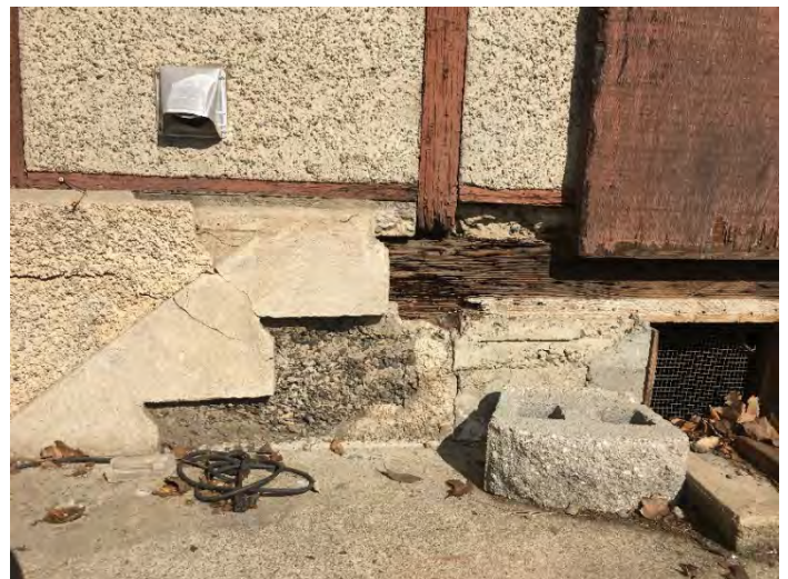
Figure 12: Deteriorated sill plate at former basement stair location.
