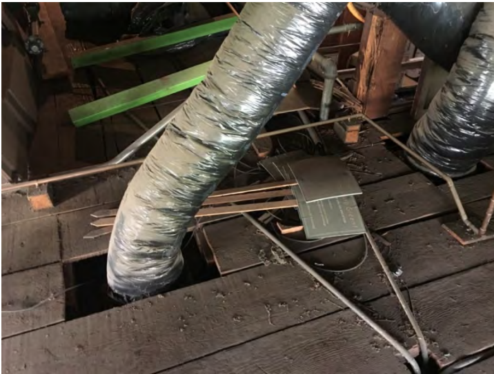
Figure 90: Supply air provided through openings in attic floor
