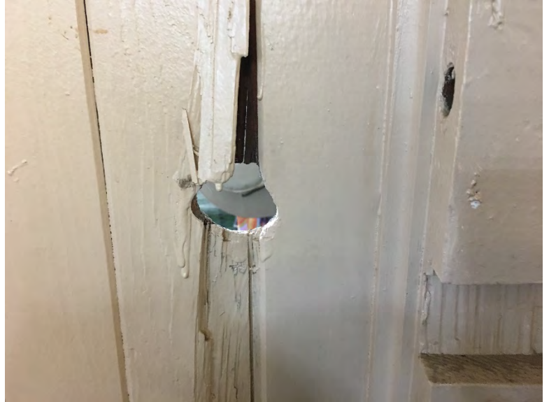
Figure 57: Tongue and groove partitions are one layer thick as this damaged partition indicates. The courtyard is visible through the hole.
