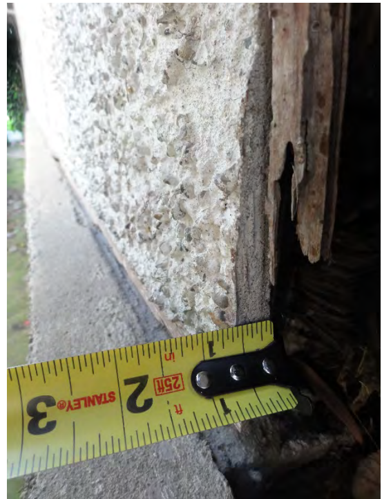
Figure 18: Thickness of exterior cement plaster panels
