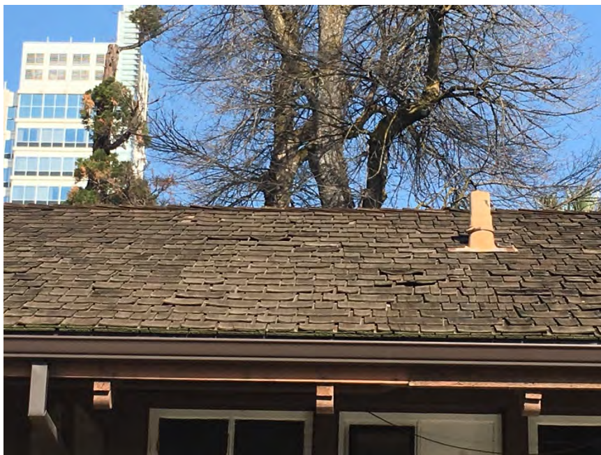
Figure 104: Plumbing vent can be seen at the roof
