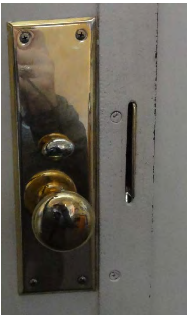
Figure 80: Entry door knob and night latch
