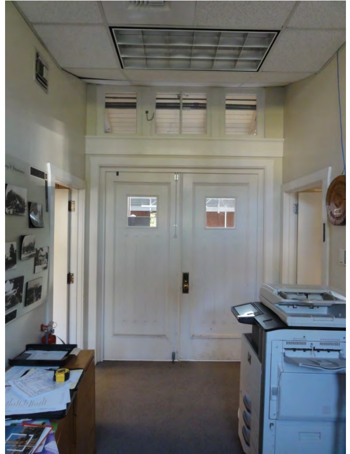
Figure 70: T-bar ceiling in main entry
