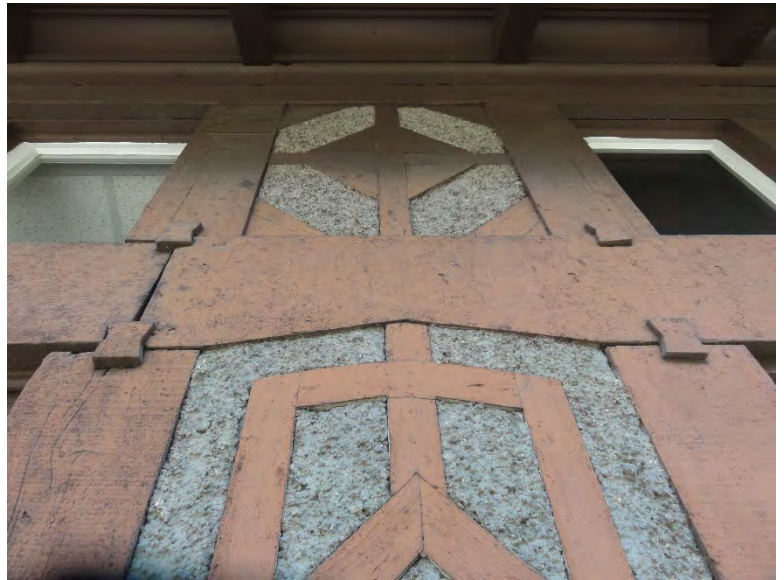
Figure 49: Redwood mortis and tenon detail at the west facade
