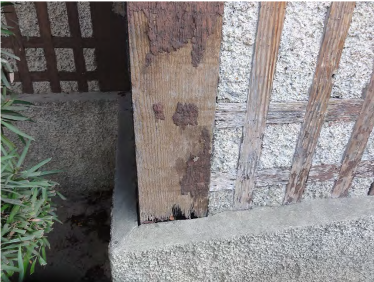
Figure 17: Base of redwood post showing water damage
