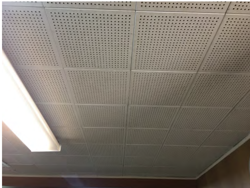
Figure 71: Drilled acoustical ceiling tiles
