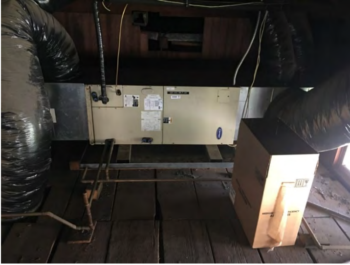
Figure 88: One of two attic mounted fan coils with insulated flex duct
