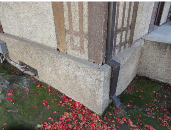
Figure 11: Northwest corner of the building showing perimeter concrete foundation
