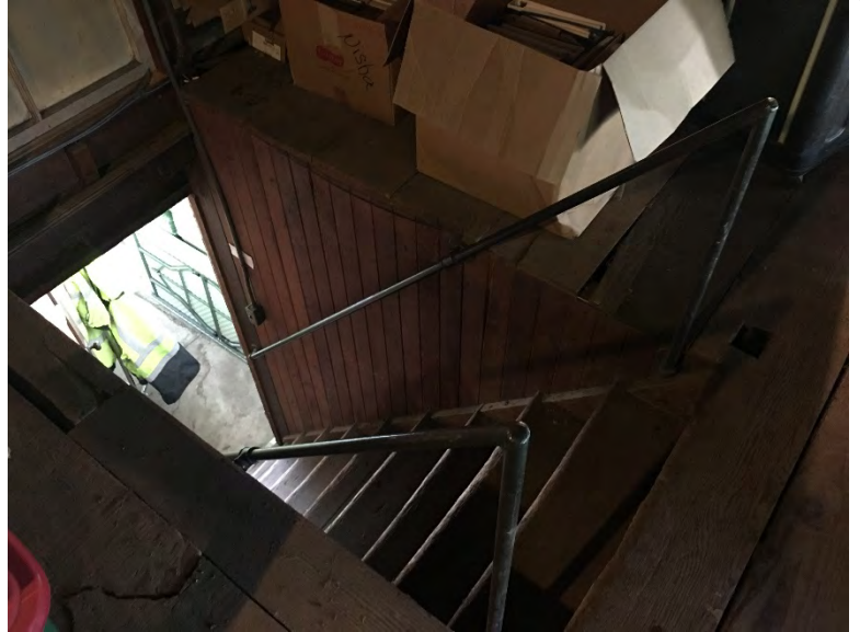
Figure 54: Attic stair, showing pipe handrails
