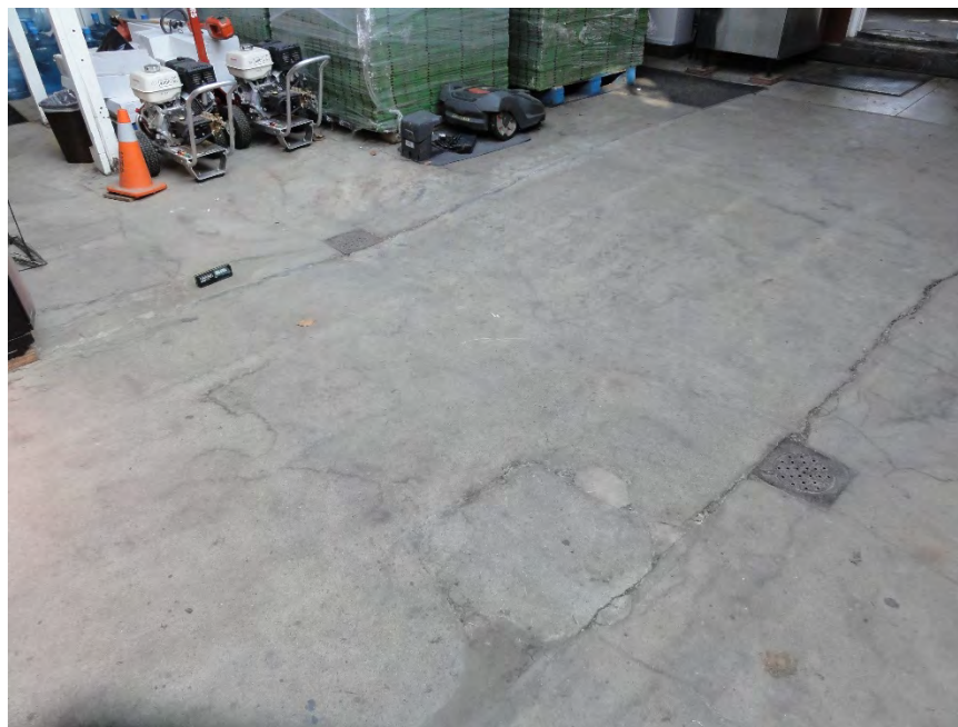
Figure 55: Courtyard floor slab sloped to drain to original floor drains.
