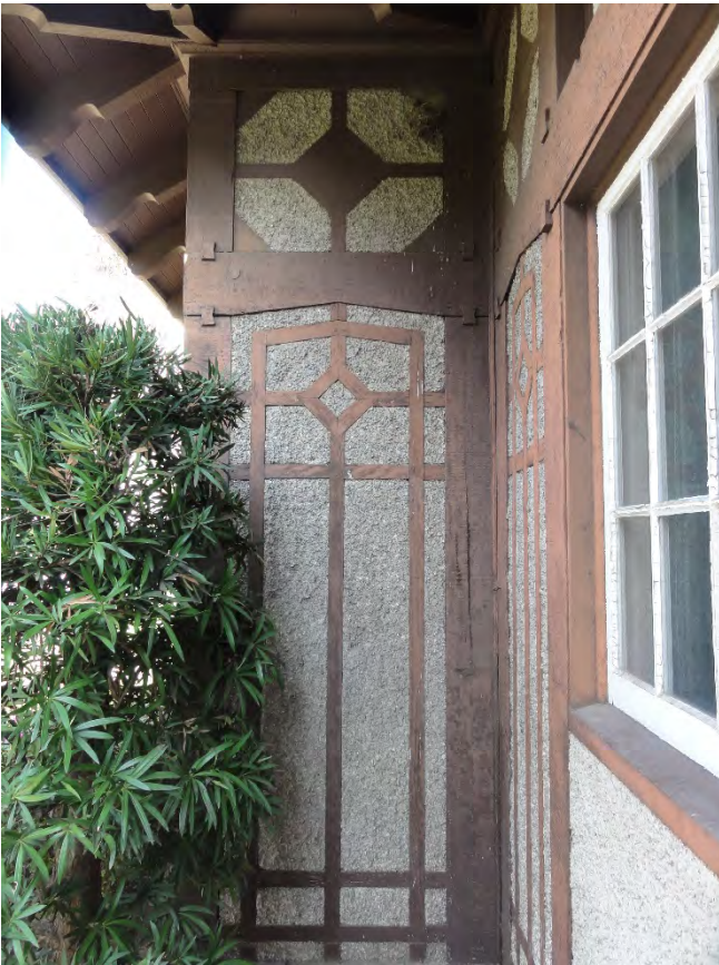
Figure 48: Redwood half-timbering exterior detail at projecting entry bay
