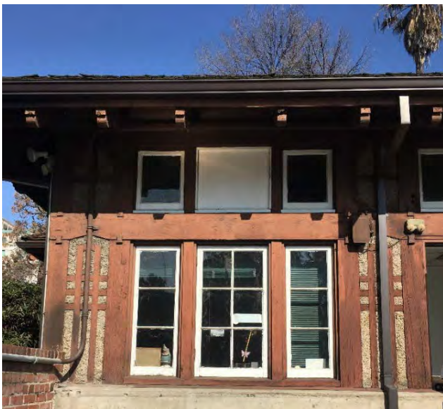
Figure 30: Typical three-part window with fixed panels at both sides and casement in the middle
